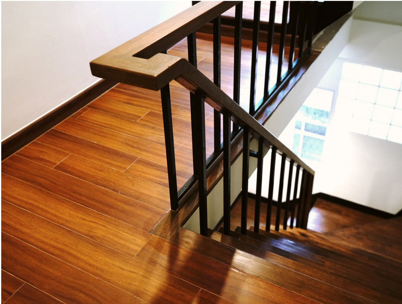
STAIR / AFTER RENOVATION
