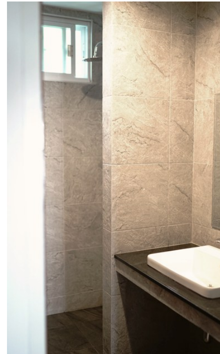
BATHROOM / AFTER RENOVATION
