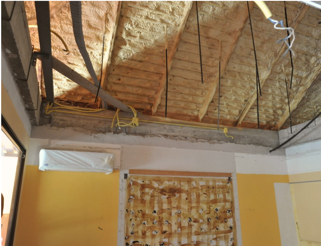
CEILING &amp; SERVICES / SITE PHOTOGRAPH
