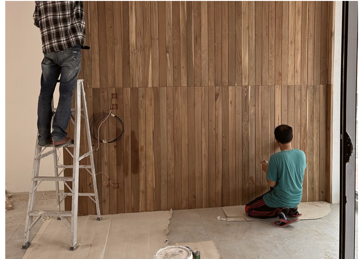
TIMBER LINING / SITE INSTALLATION
